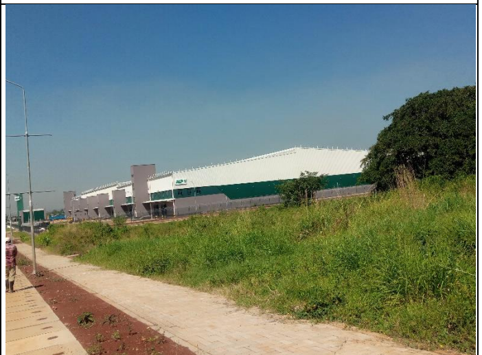
Completed Facility for Africa Logistics Properties on the south eastern border of the Project Site
