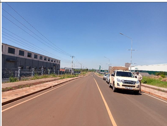
Another Facility Constructed opposite the Project Site; electricity and Road available
