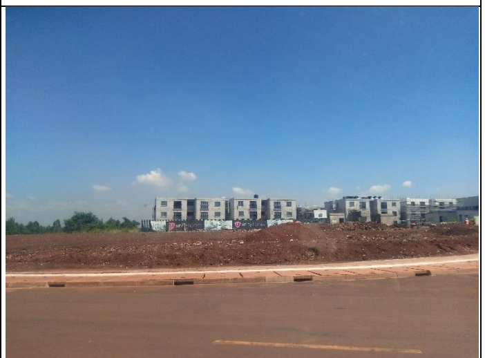
Ongoing construction activities in the wider Project Area
