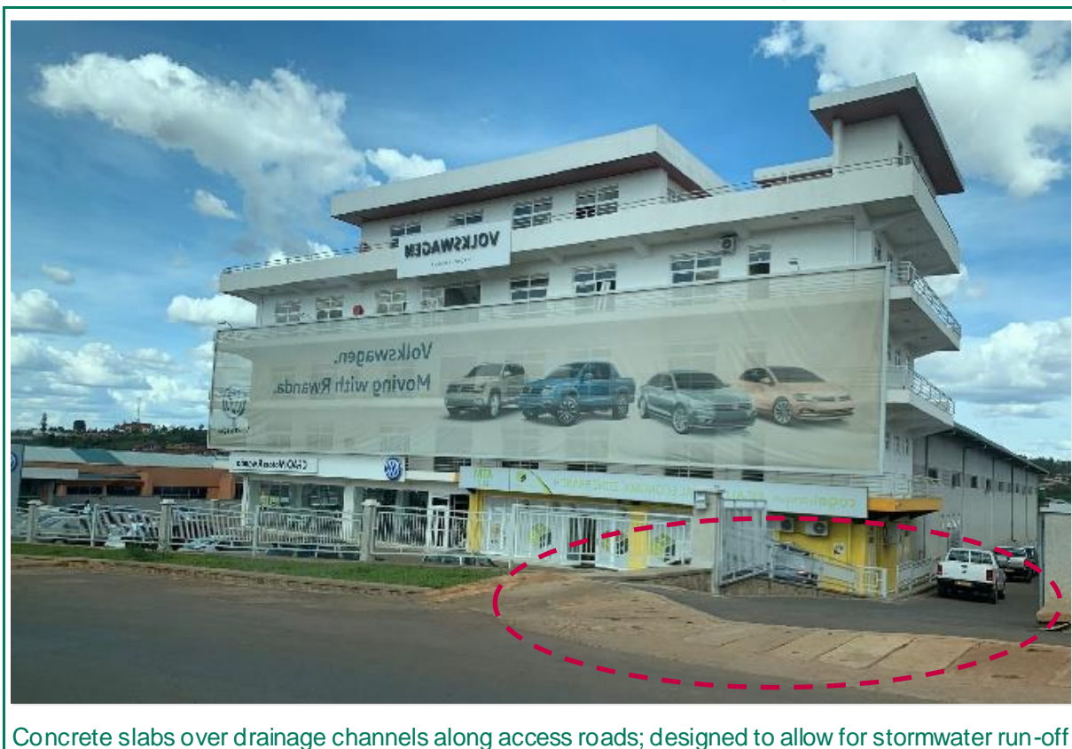
Figure 7-3 Water Management Infrastructure within the KSEZ
