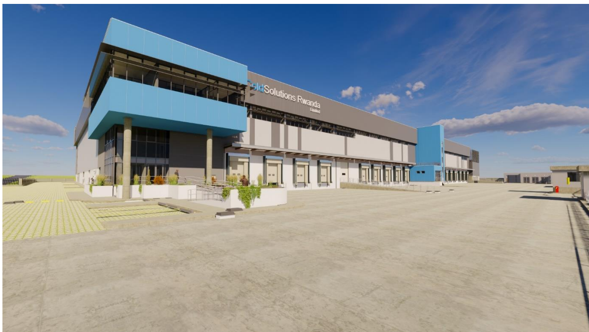
Figure 4-3 provides conceptual layout of the Project facility including the superstructure and docking bays.
